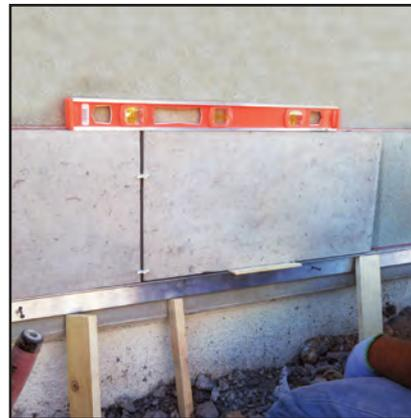
Using a propped up rigid aluminum channel can help you support and level out the first row of tiles during installation.
