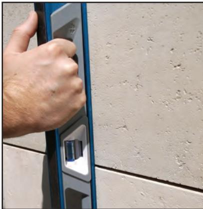
Use a large level to check and maintain an even-face plane over multiple tiles.
