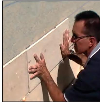
Work the stone into the wall using a left-to-right motion until mortar squeezes from the perimeter of the tile and full-coverage adhesion is achieved.
