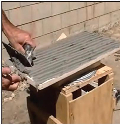
Use a 1/2" notched trowel to apply non-sag thinset bonding mortar to the back of the stone.
